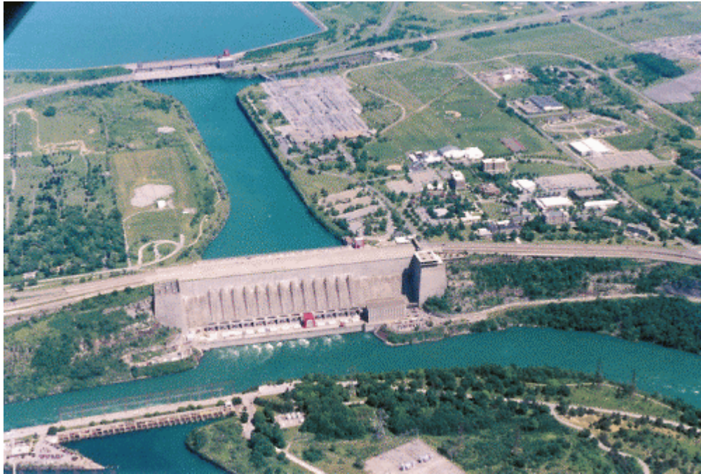
Figure 7. Lewiston reservoir (top), Robert Moses Power Station (middle) and Sir Adam Beck Power Station No. 2 (bottom left) along the lower part of the Niagara River. [7]
